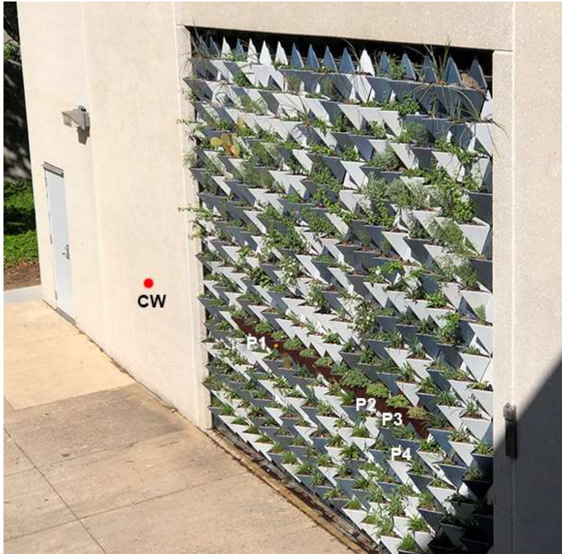
Figure 2. Image of the MLWS at noon, June 22, 2022. Locations of P1, P2, P3, P4, and CW are shown. Vegetation (P1- C. lanceolata ‘Sterntaler’, P2- A. millefolium , P3 - L. muscari , and P4 - O. speciosa ) were selected for their moderate water needs, canopy cover, and leaf and floral interests.
