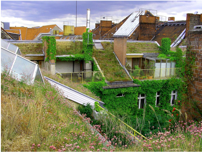
Figure 5. The PLU (Paul-Lincke-Ufer) roofs today: the green roofs are well developed, and the climber has covered all the facades. All areas are in good condition and will thrive for years to come.
