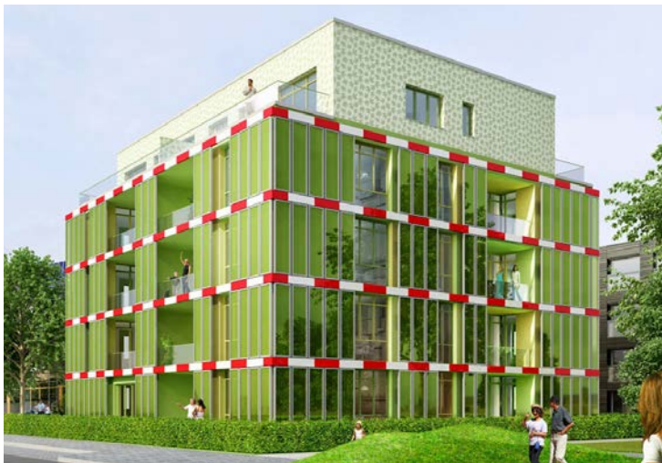
Figure 4a: The BIQ House in Hamburg, Germany, features an innovative bioreactor façade. Photo: Arup
