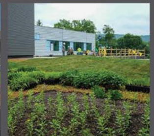
SUNY Cobleskill Cobleskill, NY Semi-Intensive Green Roof
