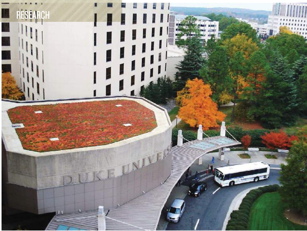
TOP: Duke University Health System green roof Image provided by: Duke University Health System
