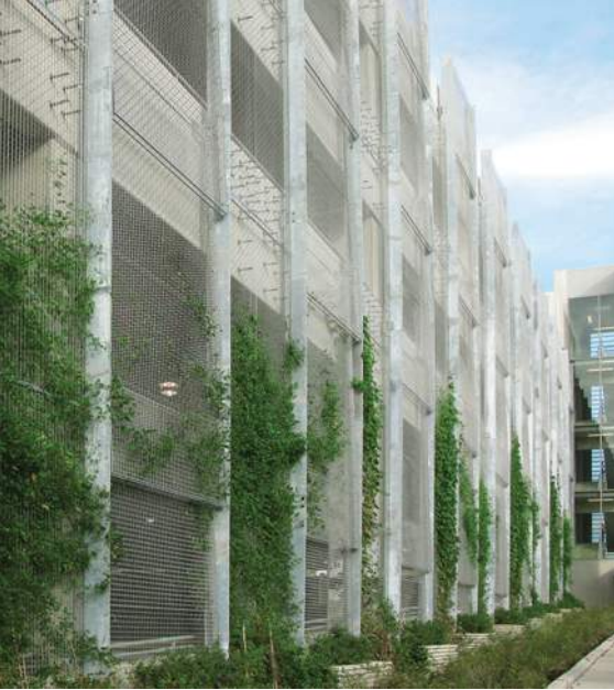
THIS PAGE: Staten Island Courthouse parking structure green facade before & after Sandy (top, before / bottom, after) Image provided by: greenscreen®
